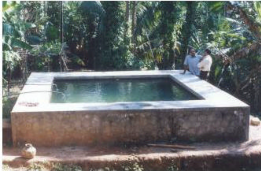
Plate-5 Storage tank (concrete) used for both domestic & irrigation purposes
