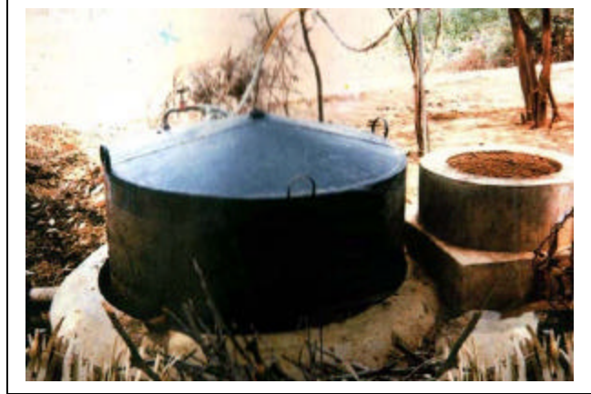
Fig: 5 Gas Holder filled with gas in KVIC Plant- gas holder floats above the ground level
